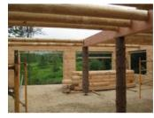
structed and the LVL ridge beam raised into place. Once the conventional 2X10 rafters were in place, 2X4 purlins were added and a "green board" before the metal roof panels were secured. Open celled "soy" expandable foam was sprayed
