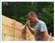
the pre-cut 8x12 into place. Once Curt's homegrown post was in place, pre-cut log floor joists were dropped into the wall and girder pockets and secured. Another three courses of logs were added for the knee-wall before the gable ends could be con-
