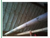
from inside between the rafters to keep any air from entering the roof system and to provide an R-40. Recycled bluejean batts were used to provide the insulation for the first floor before the fire-code drywall was added to the basement garage area ceiling.
